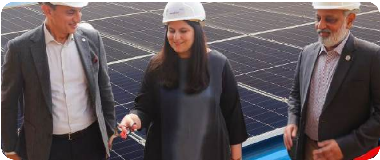
Commissioning of 1 MW Solar Installation at Sheikhpura Factory
